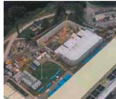
Clear Water Tank under construction
